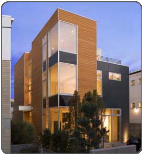
Site Pictures By: Frank Ooms Photography
