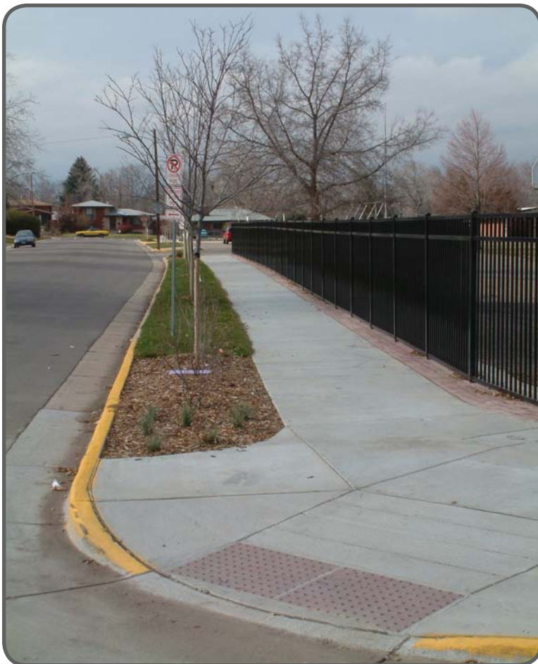
Emerald Streetscape overlooking new ADA curb ramp
