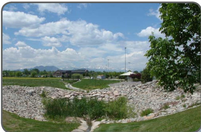
Existing pedestrian bridge overlooking downstream drop structure (top)
