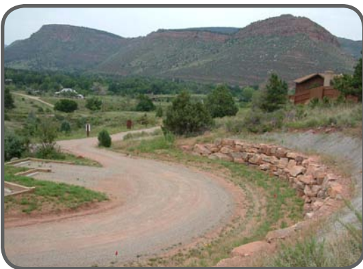
Cul-de-sac parking overlooking drystack wall
