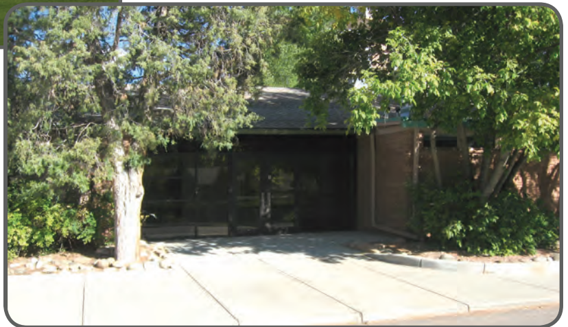
Modified ADA entrance to Lyons Elementary School
