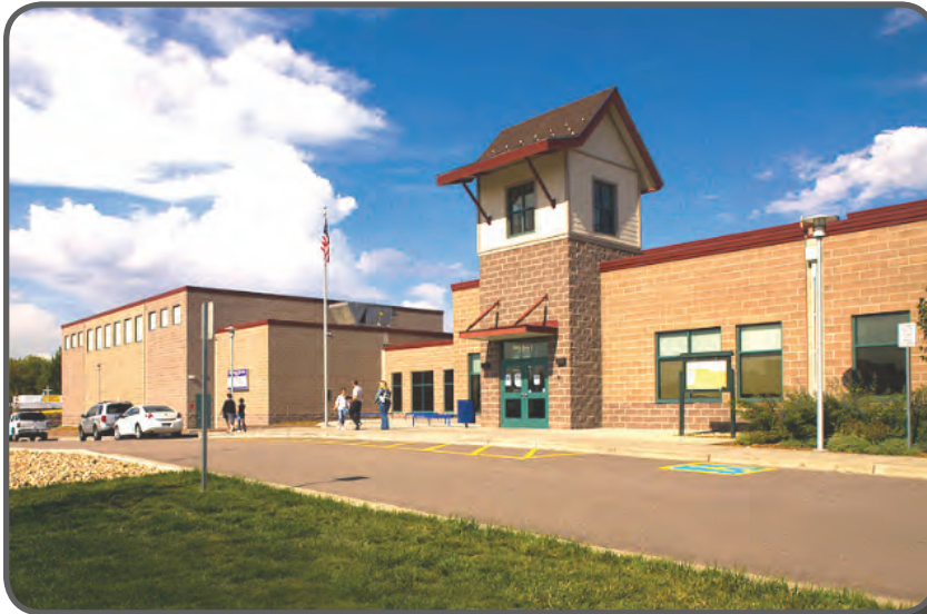
Front of school and new gymnasium overlooking
