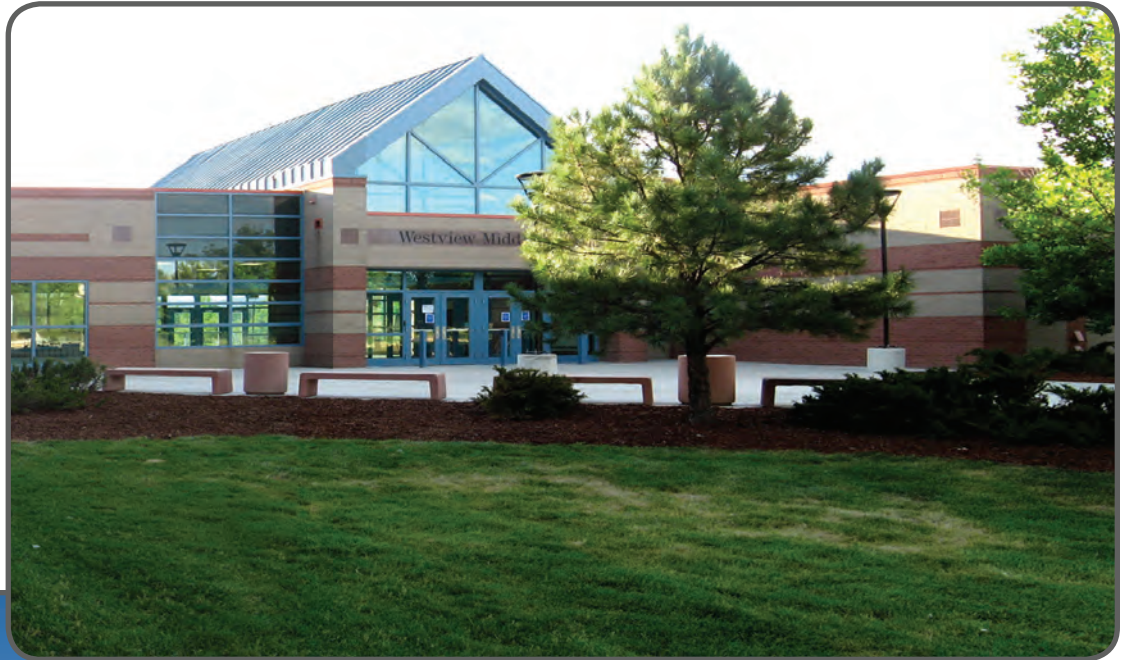
Modified front entrance and courtyard
